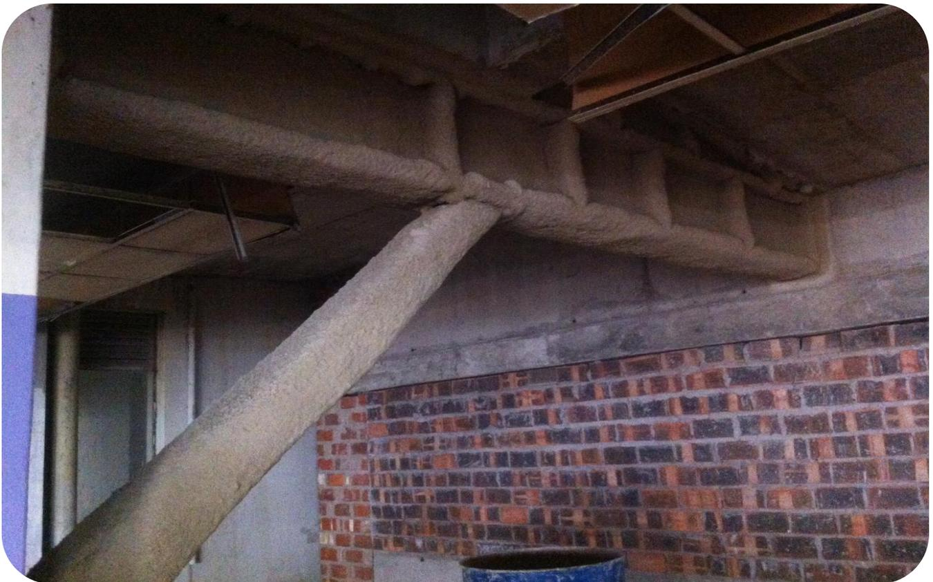
A photograph of a recent fire protection in the Cape, the requirement was to provide a 2 hour fire rating at the most economical rate, in order to do this the product submitted was Tekrok S a low density fire proofing plaster supplied by Mandoval Vermiculite CC an ISO 9001:2008 accredited company.
